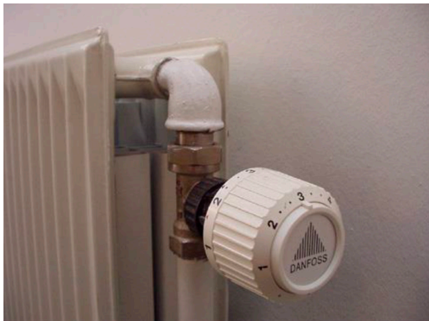
Figur 19. Radiatortermostatventil
